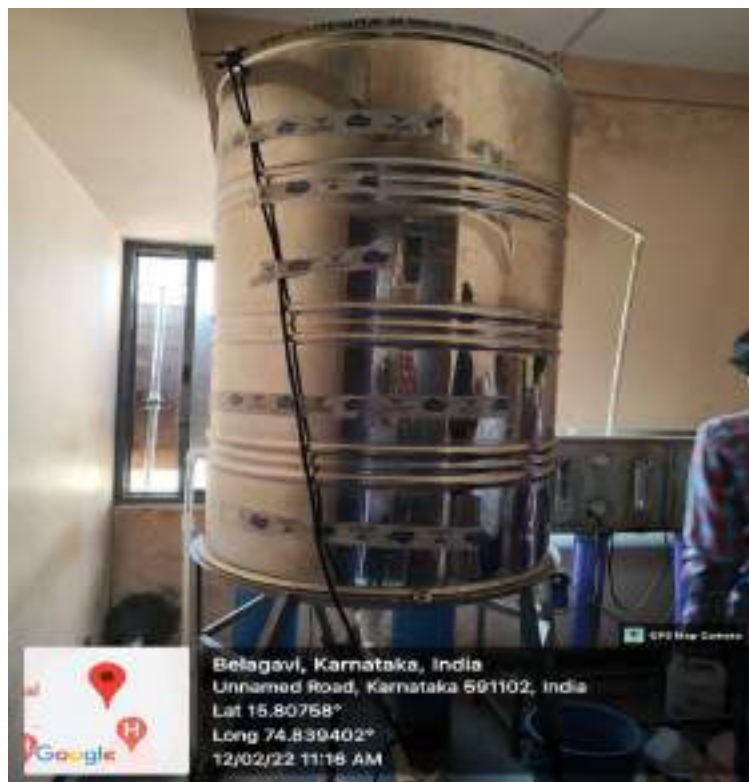
Drinking water storage tank at college canteen
